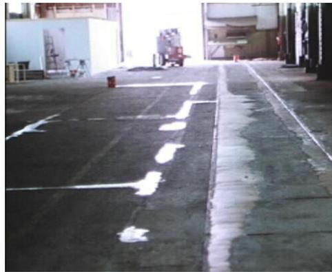
The photo shows a close up of the steel rail cover by ShurBond 500. The photo on the right shows one of the rail lines after smoothing with ShurBond 500. The area to the left shows concrete failure areas that have been repaired with ShurBond 500.
